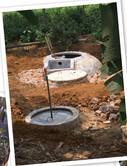
Helping the neighbours instal a bio gas unit
